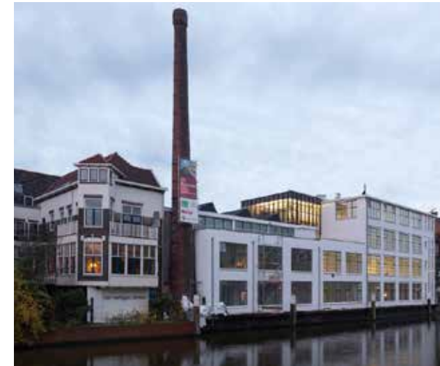
Figure 2. “De Fabriek” building
