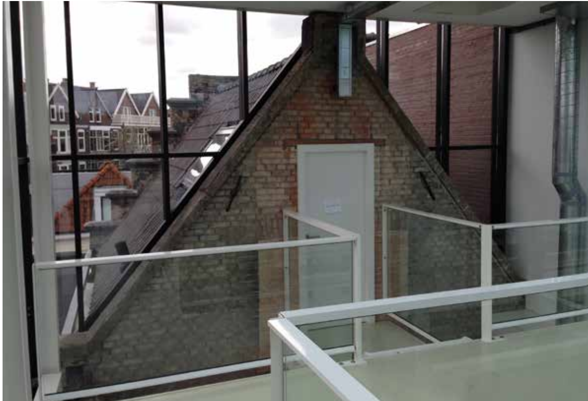
Figure 5. Connection between old and new in "De Fabriek"
